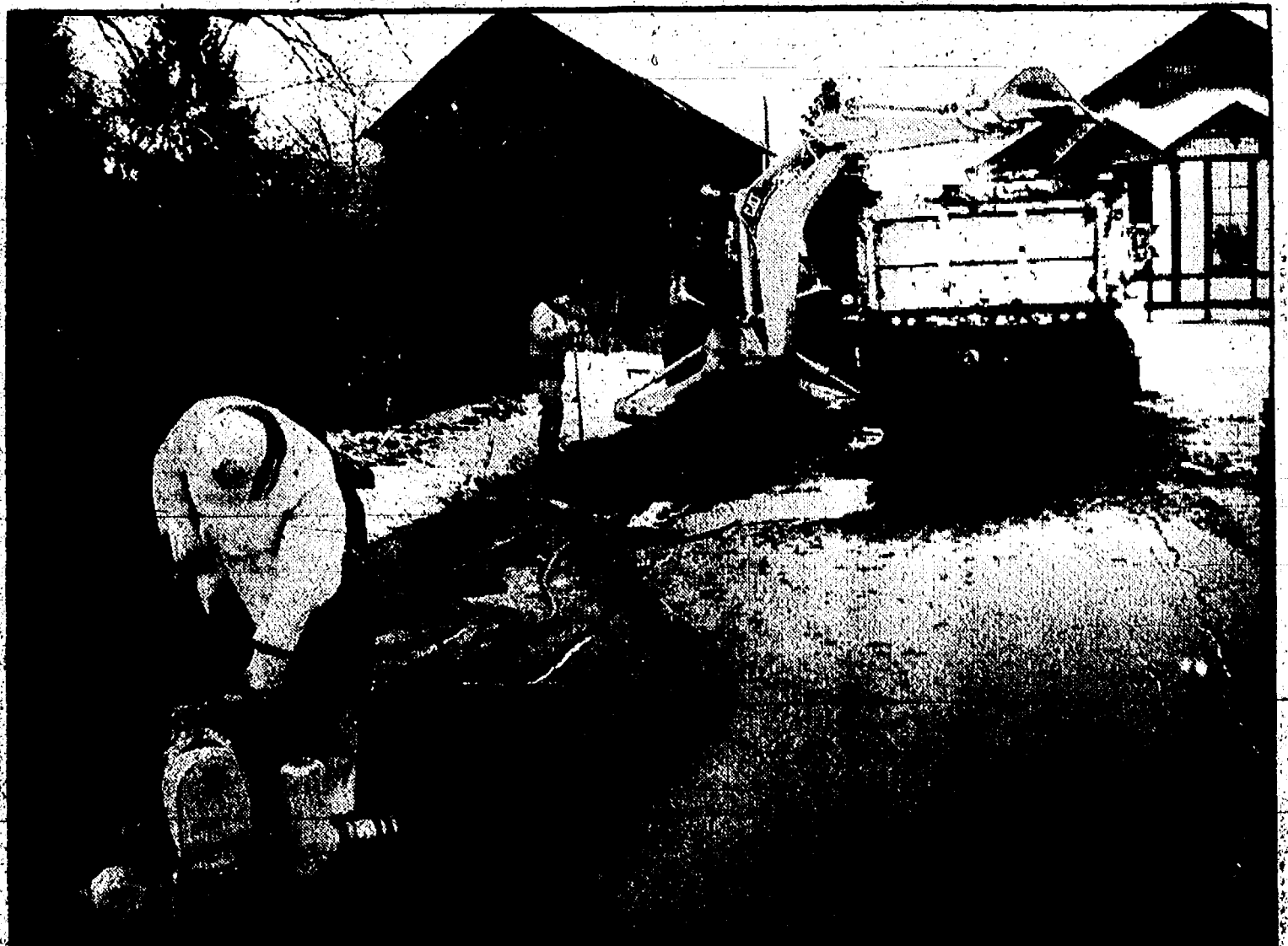
A WATER MAIN broke over the week-end on Jackson Street next to the Chelsea Depot, a fairly common occurrence during the coldest months. The street had to be closed off while workers pumped out the water, excavated the site, and fixed the problem.
